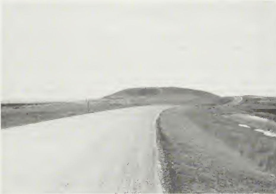
Figure 8 - South view near milepost 14.7
